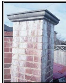
Watertight mortars and concretes obviously protect the underlying substrate better and last considerably longer than those, which are porous – especially in salty atmosphere marine locations.
